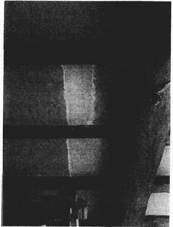
Ceiling fire boarded / repaired
